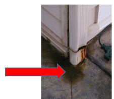
Fencing is in in bad shape. The original builder used 'builder spec' materials that were the minimum for the job, but these materials were not of the quality needed to resist rot and are now in need of significant repairs. Fence pickets are rotting and missing, and many of the untreated posts are rotting at the base and will need to be replaced. Vinyl fencing would have much longer life and not require painting.
