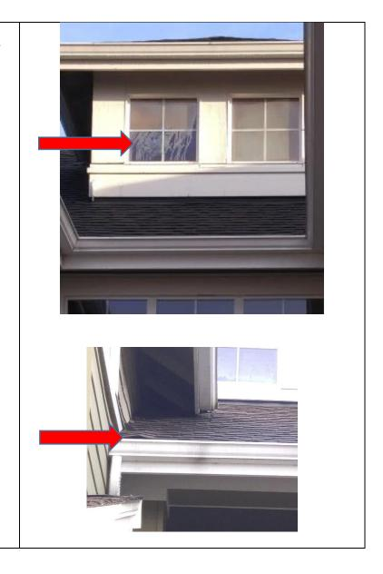
There are a number of problems with gutters and downspouts that require repair as they are spilling water onto siding and trim and causing decay
